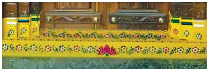
Fig 1b: Carved entrance door with yellow paint as it indicates haldi (turmeric).
