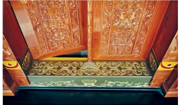
Fig 7: Main doors with brass threshold
