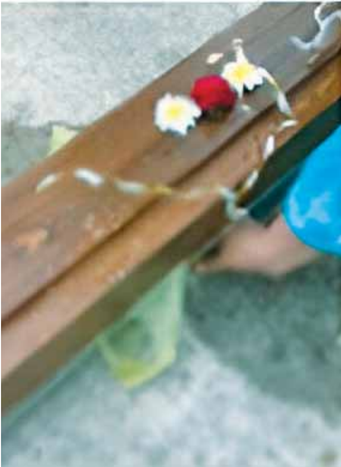
Fig 5: Fixing of door and threshold pooja and placing panch dhatu below it.
