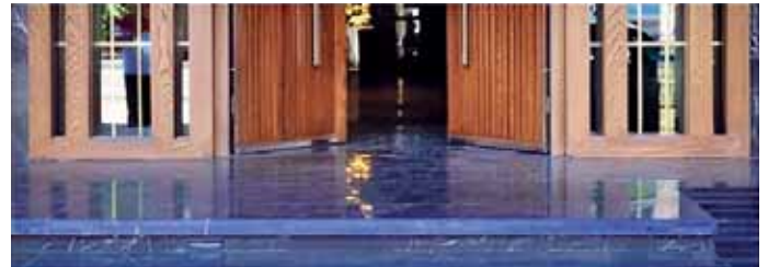
Fig 9: Modern entrance door without threshold
