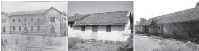
Figure 2: City High School 1853-54, 1870 & American Mission: Early School Buildings Source: Kulkarni, 1953
