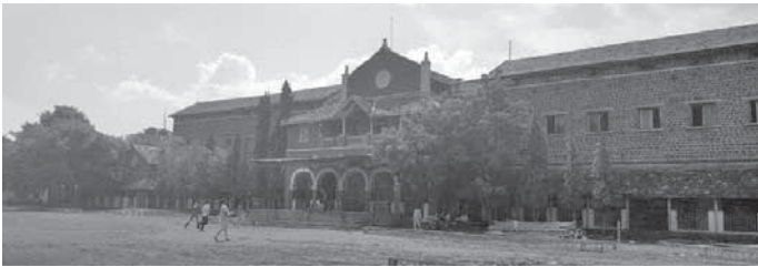
Figure 6: Northcote High School: Eastern (Rear) View Source: Author
