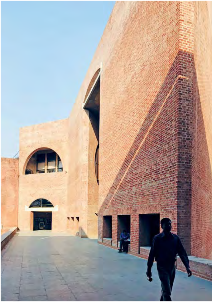
Figure 1: Long Span Corridors at IIMA Source: Author
