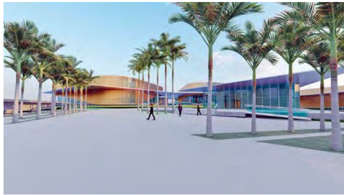
Figure 9: Administrative Block Source: Author, 2024
