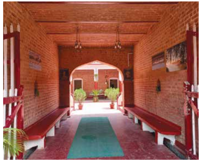
Figure 1: Architectural elements - tudor arch, niches and jack arch roof Source: Author
