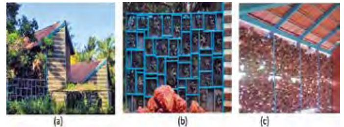
Fig. 2: Skin and Bone Residence (a) The structure (b) Car radiator fan façade (c) Coconut shell wall Source: Author
