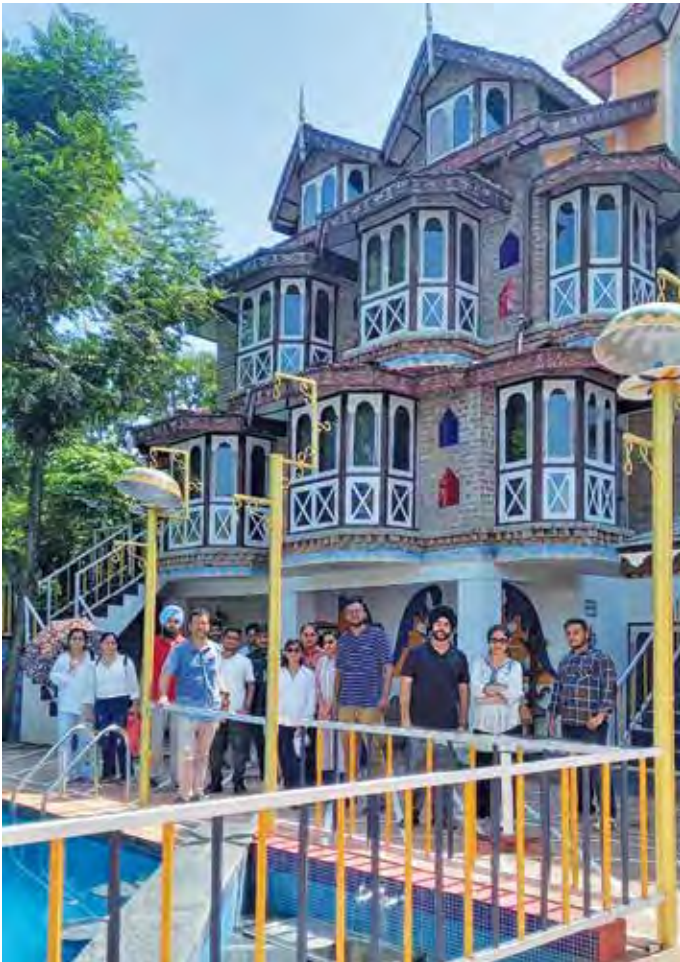
Figure 10: Colonial, Portuguese, Mughal, Rajasthani and Kangri styles of architecture at Chateau Garli
