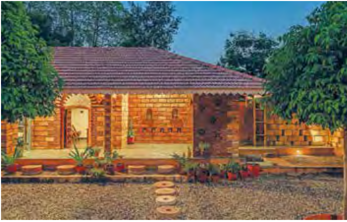
Figure 6: Architect's Office Source: Ar. Himashu Patel, Inclined Studio
