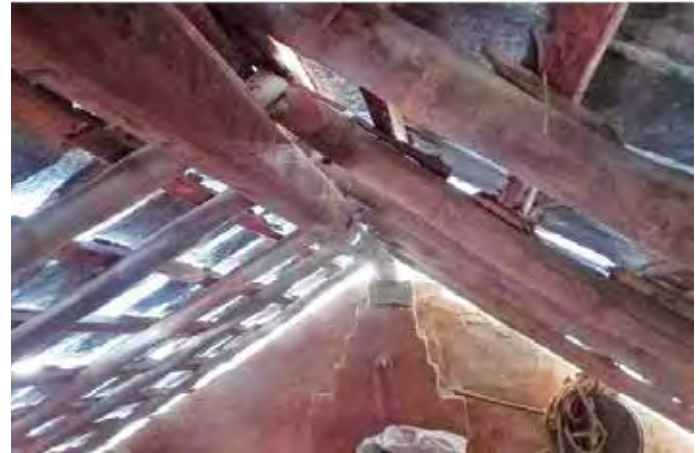
Figure 4: Vernacular construction details with wood, mud and slate shingles Source: Author
