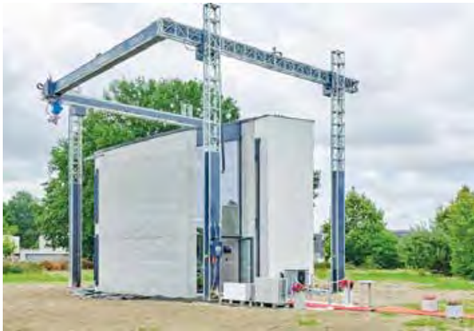
Figure 2: Curved walls produced by BOD2
