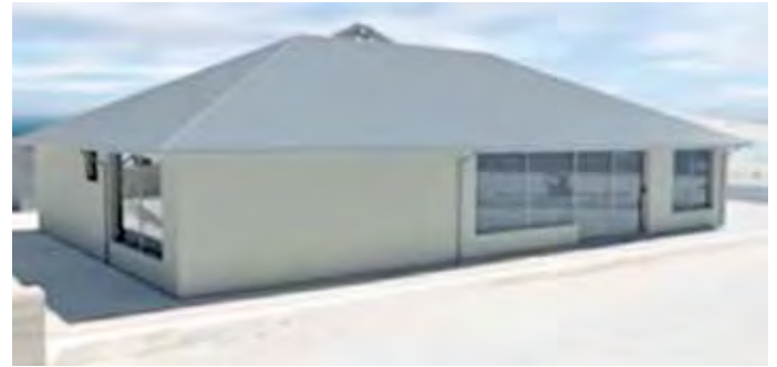
Figure 6: The finished structure by Hadrian X in less than 3 days
