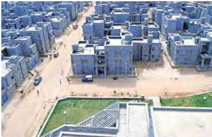
2. Aerial view of Jal Vayu Vihar
