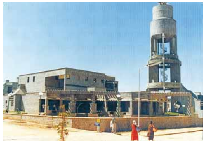
7. Water tank and multi-functional hall
