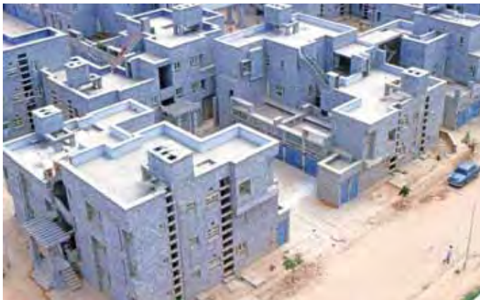
3. Aerial view of Jal Vayu Vihar
