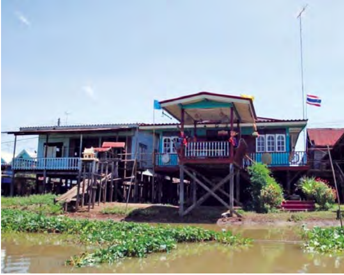
Fig. 2: Traditional House along a khlung (canal) in Lat Chado, Ayutthaya Province, Thailand Source: Author
