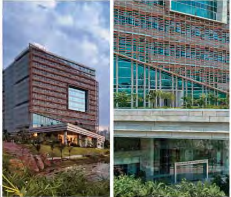
Some portions of the façade do not have a second skin and are inset by 2m into the building for glare and heat protection
