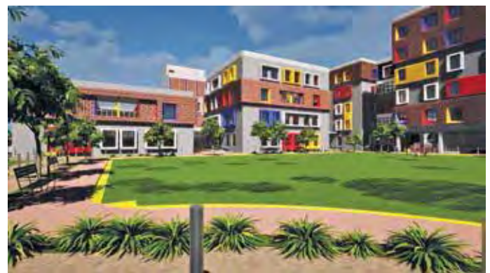
Figure 15: A view showing the arrangements of building blocks in an ascending order
