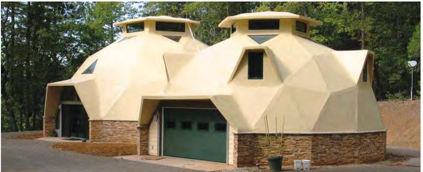
Fig. 6: Geodesic Dome-Shells with Concrete Panels
