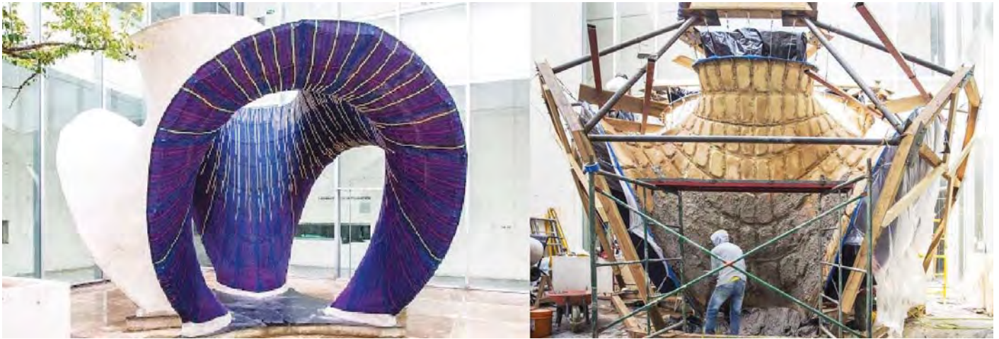
Fig. 8: Knit Candela shell: Finished and Under-construction
