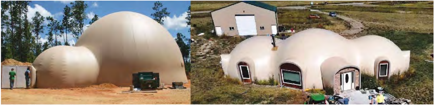
Fig. 7: The inflated Airforms & a complete Dome House by Monolithic Domes
