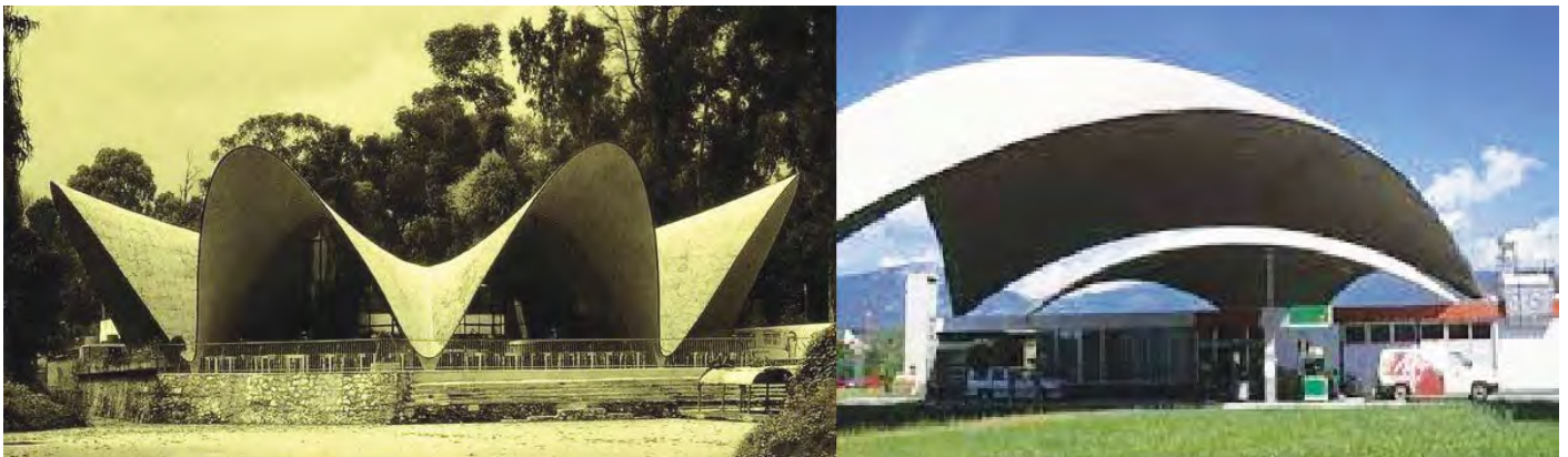
Fig. 2: Los Manantiales & a concrete shell by Heinz Isler Source: David P. Burger (2006) & Heinz Isler archive
