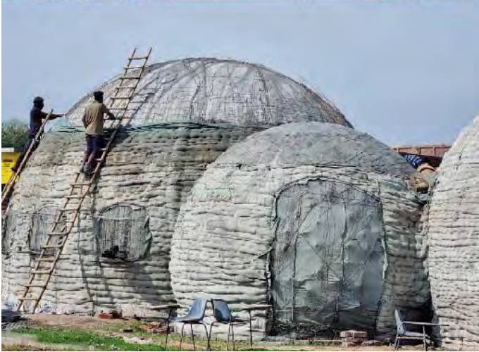
Fig. 9: An example of Radial Formwork and casting of the composite shell by Spur D Source: Author
