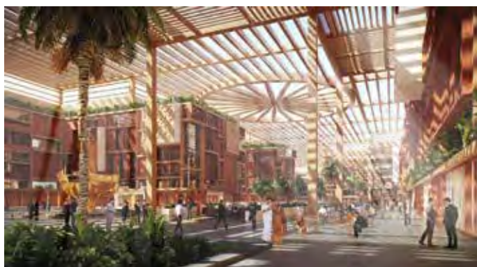
The courtyards in the secretariat buildings are shaded through pergolas, whose members are arranged to form an Ashoka Chakra.
