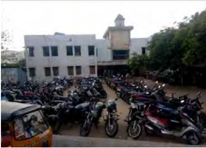
Fig. 3: Defunct entrance block (Source: Author)
