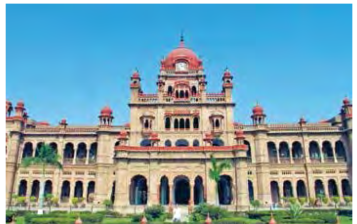
Figure 1: Front Facade of Khalsa College, Amritsar Source: https://twitter.com/moomjamma/status/1092272237787402240/photo/2
