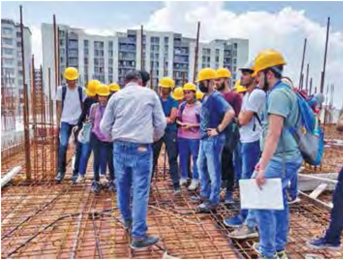
Fig. 3: Students learning about site and construction
