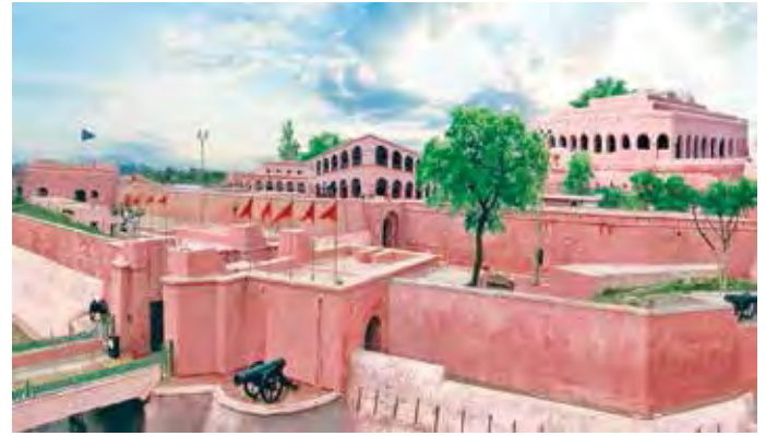
Figure 9: Restored structure of the Gobindgarh Fort, Amritsar Source: https://amritsartourism.org.in/gobindgarh-fort-amritsar
