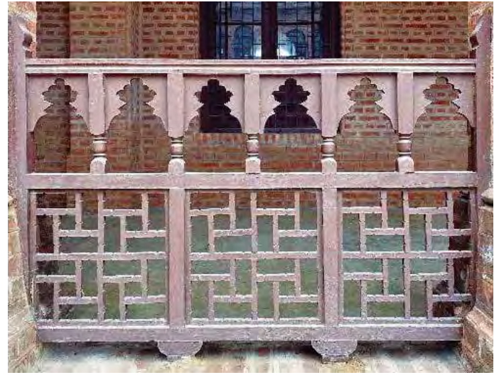
Fig. 4 : Traditional geometrical lattice work in the railing design in Khalsa College, Amritsar, Punjab Source: Corresponding Author
