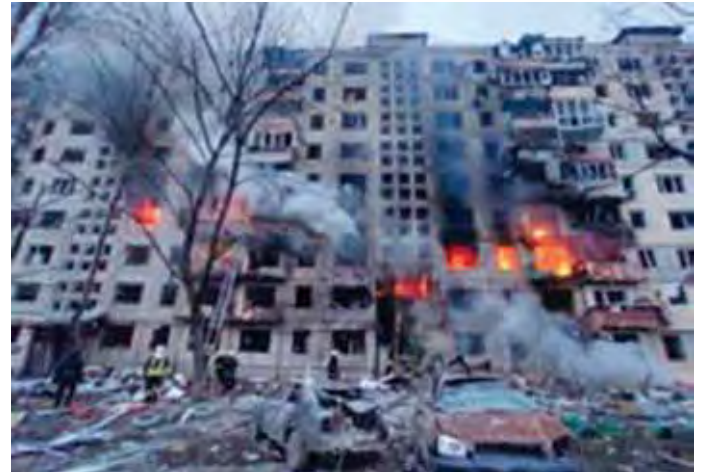
Fig.3: High-rise apartment damaged by shelling in Kyiv, Ukraine on 14 March 2022 (Source: Retrieved, January 15,2023 from https://www.reuters.com/ )
