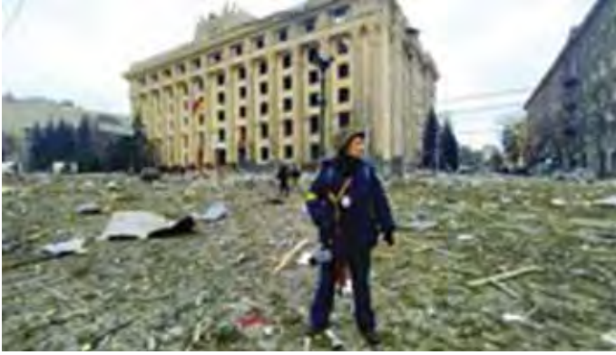
Fig.8: Kharkiv State Administration building destroyed by Russian missiles mothballed.
