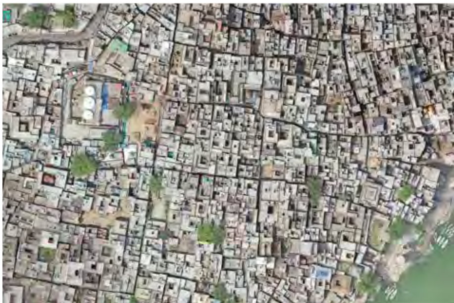
Drone shot from before work on the corridor began
