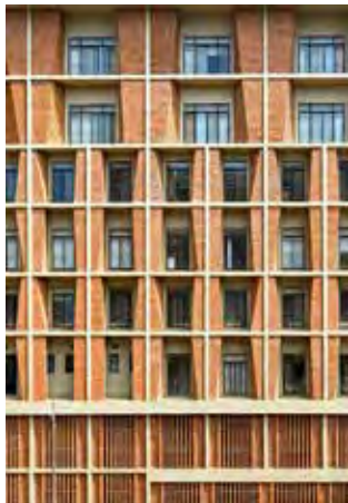
Figure 6(b): Twisted CEB boxing seen on the facade, SUHRC, Lavale, Pune (Photo Courtesy: Rajesh Vora)
