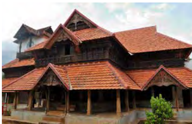
Figure 2a: Traditional houses (Source: https://www.caleidoscope.in/wp-content/uploads/2018/11/Traditional-Homes-of-South-India-Kerala.jpg (accessed on 26 Jan. 2021))
