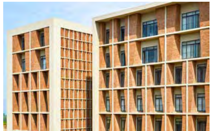
Figure 6(d): CEB jaali screens act as shading devices, SUHRC, Lavale, Pune (Photo Courtesy: Rajesh Vora)
