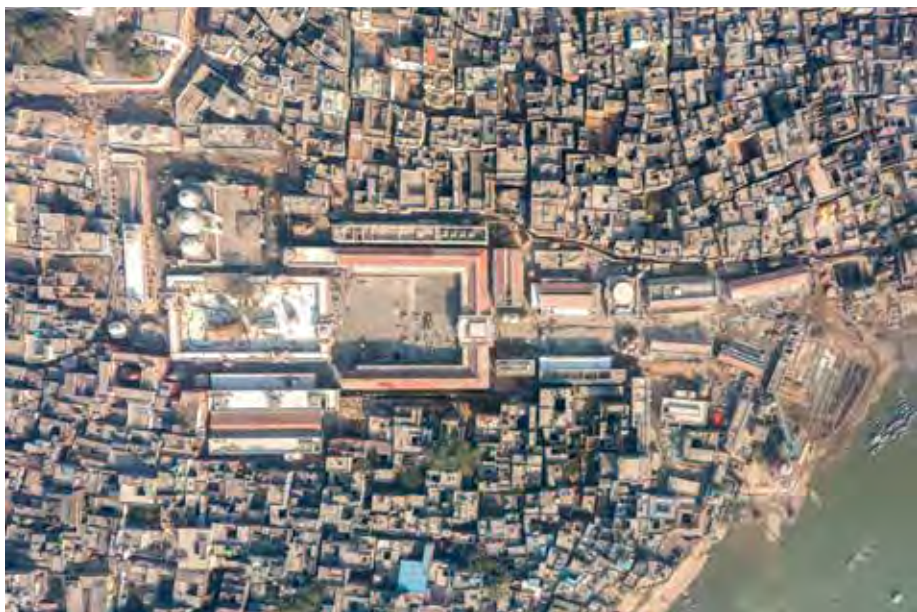
Drone shot of the project nearing completion
