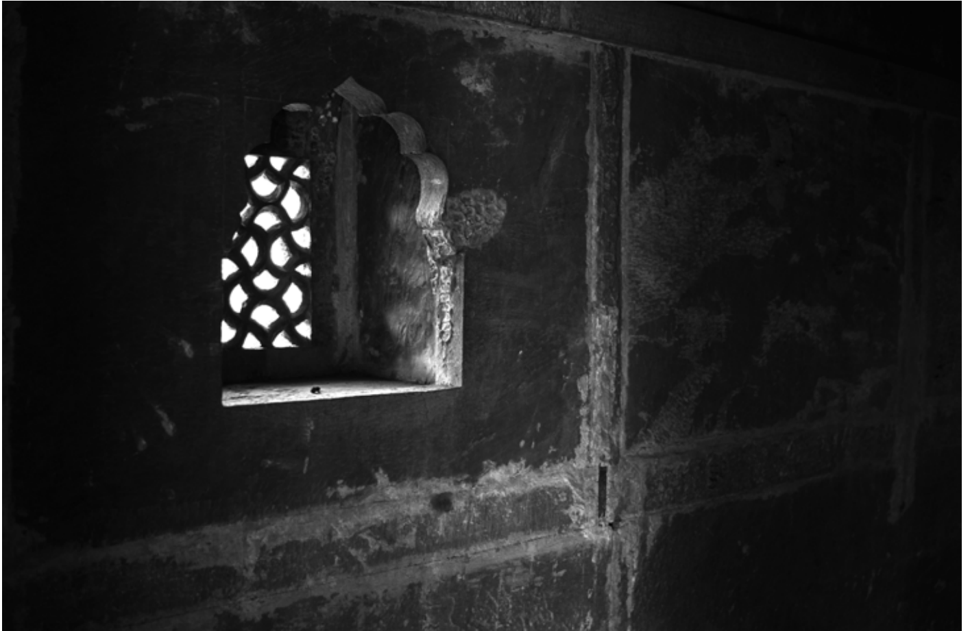
A small ventilator just about enough to make the low height 'Kop Bhawan' breathable.
