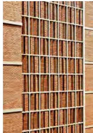
Figure 6(c): CEB jaali screens act as shading devices, SUHRC, Lavale, Pune (Photo Courtesy: Rajesh Vora)
