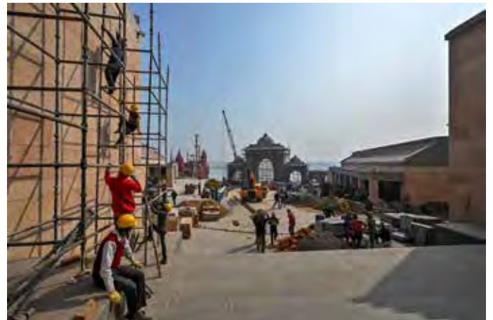
The pathway from the Temple to the Ganges, under construction
