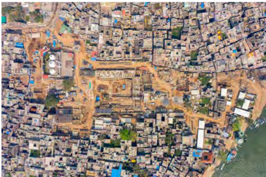
Drone shot of the project under development
