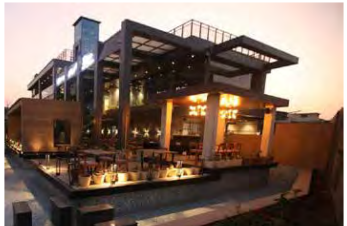
The building showcases a variety of spaces
