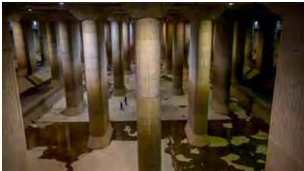
Figure 2 : Underground discharge and its floodwater cathedral (Source: https://www.tourist-destinations.com/2014/11/g-can-flood-surge-tunnels-in-tokyo.html . Accessed on 4 Jan. 2020)
