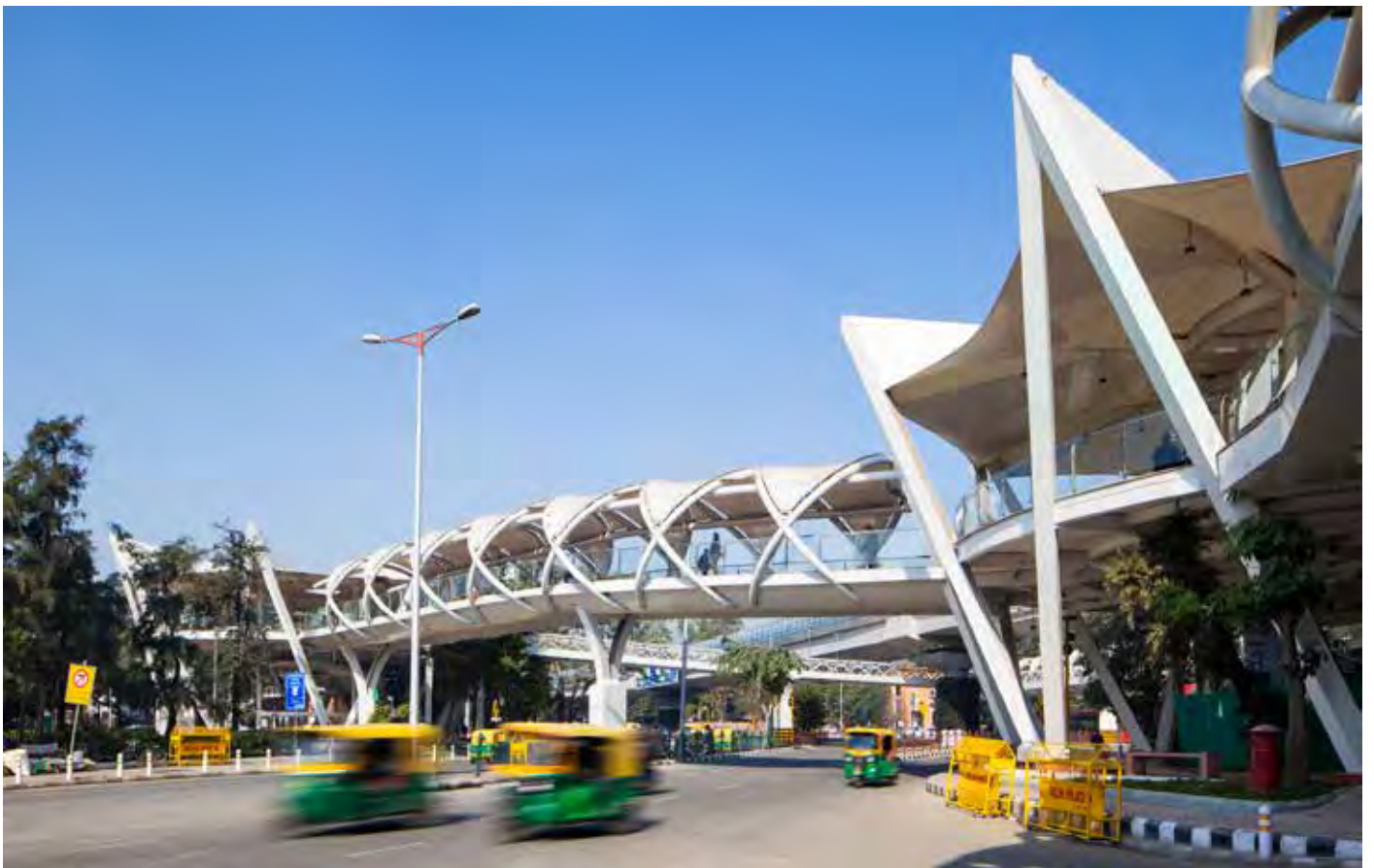
The winding walkway appears to be floating above the high-traffic junction.
