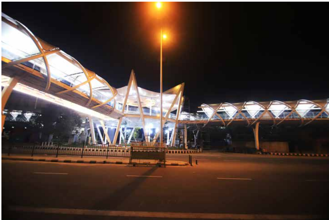
Multiple walkways come together and meet at this octagonal structure.
