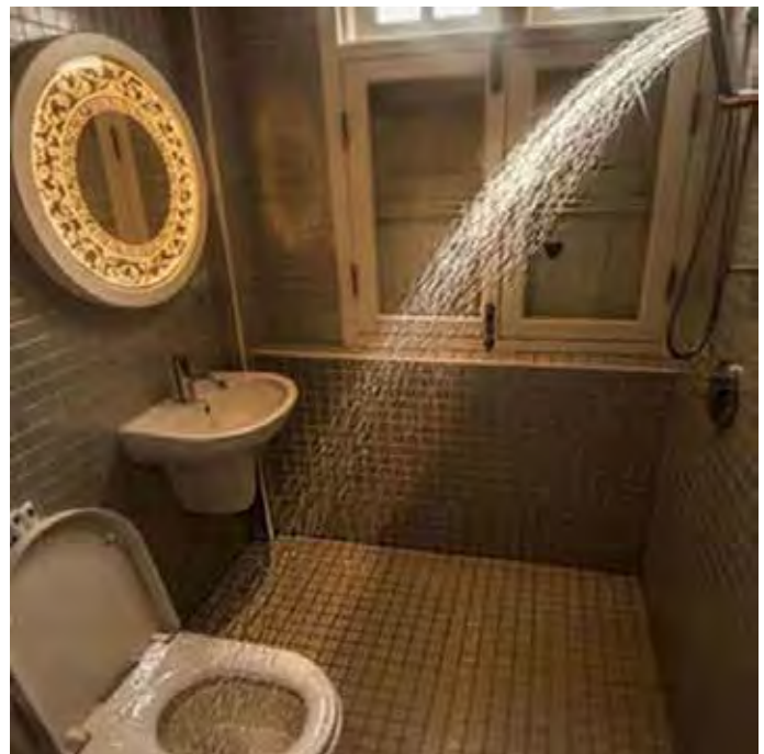
Figure 5: Position of the shower rose is such that a shower can be taken by even seating on the WC. No space for standing below the shower
