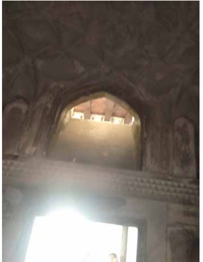
The view of the skylight from the inside, designed to facilitate wind harvesting.
