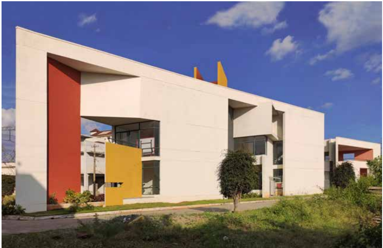
View of the Green Cascade building
