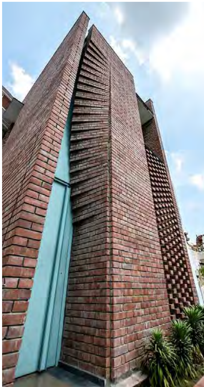
Brick Curtain Office, Karnal
