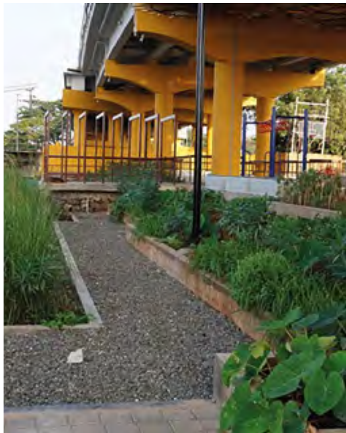
Before and after images of spaces underneath a flyover bridge in Coimbatore
