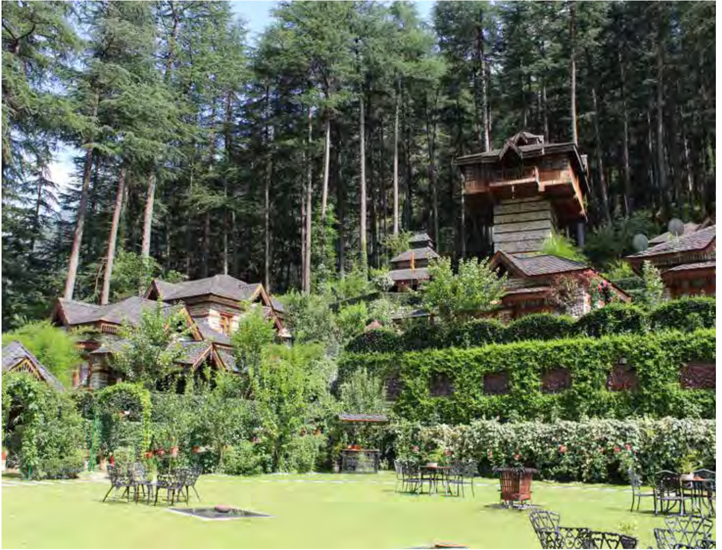
Figure 9: Dry stone retaining walls as green walls with relief work
