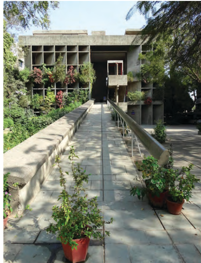
Figure 7: Mill Owner's Association Building
