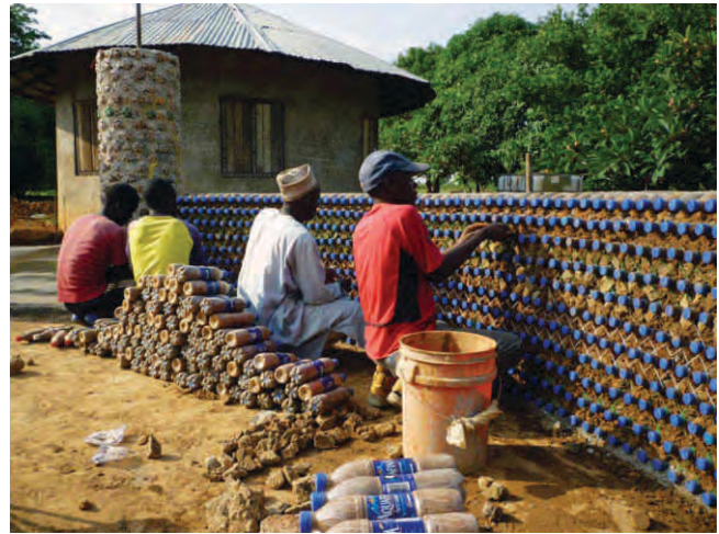
Fig-3- PET waste bottle houses in Nigeria.
