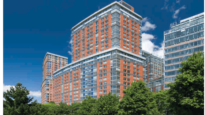
Figure 13 The Solaire, New York City
