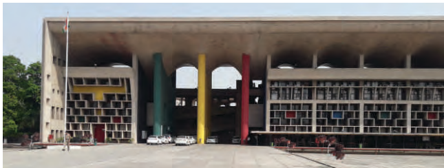
Figure #3: Brise Soleil at Palace of Justice
