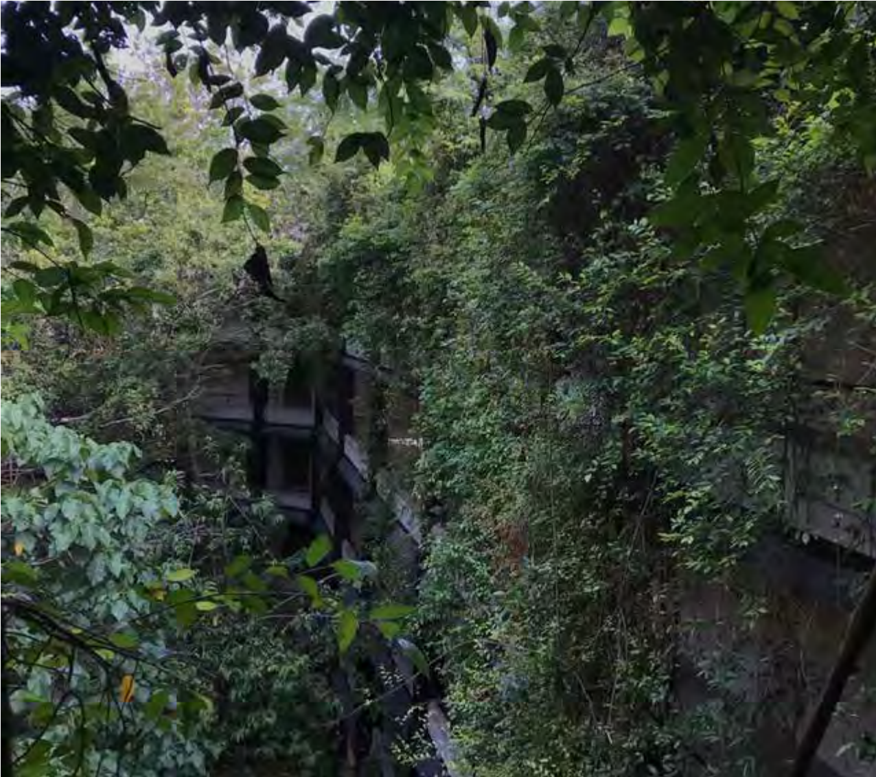
The Kandalama Hotel, is designed to be taken over by the forest context surrounding it, making it one with it, in an ongoing process of "completion" of the building.
