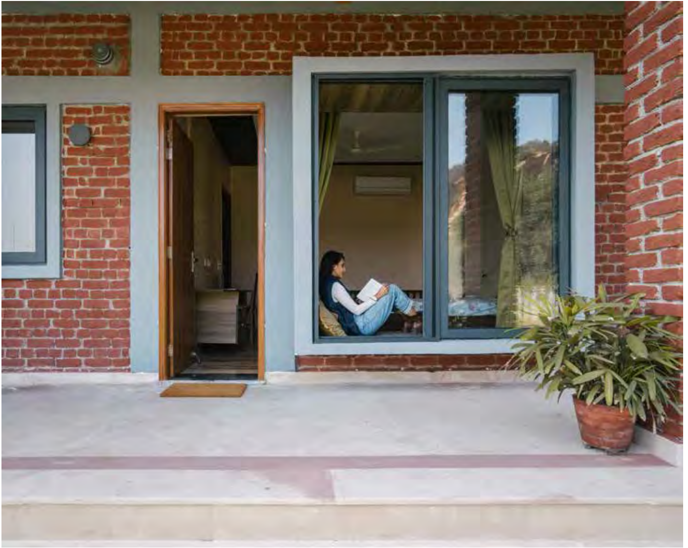
Box windows projecting onto the Verandah.
