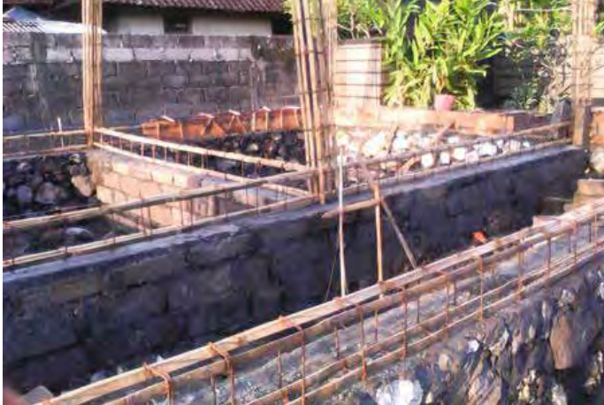
Bamboo reinforcement in plinth beams (Source: Author)
