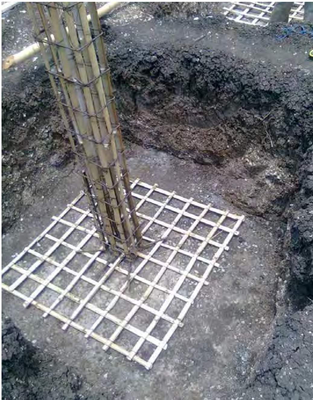
Bamboo reinforcement in footing (Source: House Owner)
