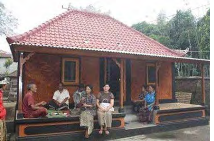
Exterior view of the G+0 structure (Source: Author)
