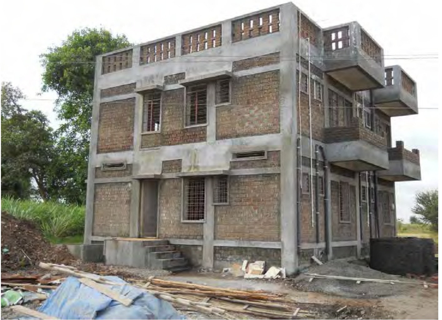
Exterior view of the G+1 structure (Source: House Owner)
