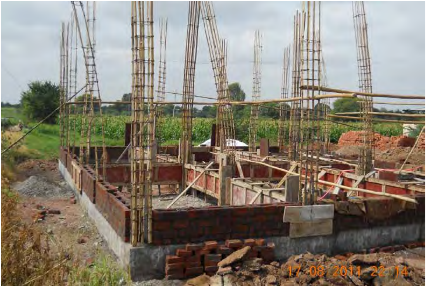
Bamboo reinforcement in columns (Source: House Owner)
