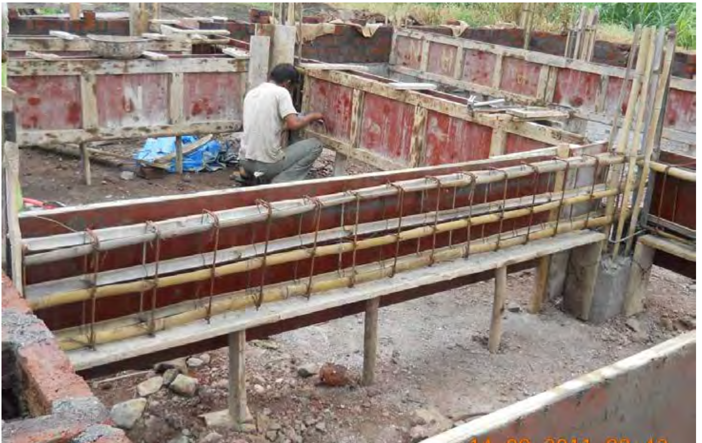
Bamboo reinforcement in plinth beams (Source: House Owner)
