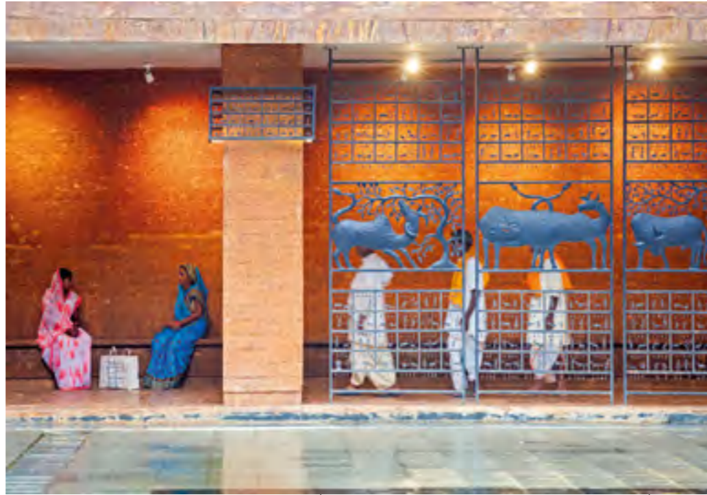
Left ► Expressed in locally-sourced laterite, the entrance to the complex opens directly into the central court.
