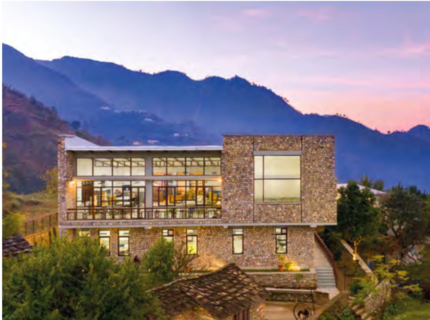
FOREST ESSENTIALS FACILITY LODSI, RISHIKESH, INDIA
