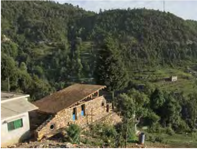
Lakdi ki Kathi - a design-and-build project in Ghuggukham, Uttarakhand
