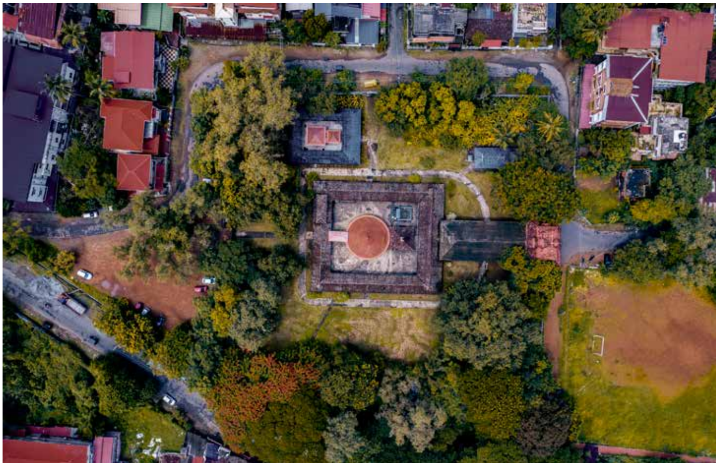
An aerial view of Punkunnam Siva temple, Thrissur District.
