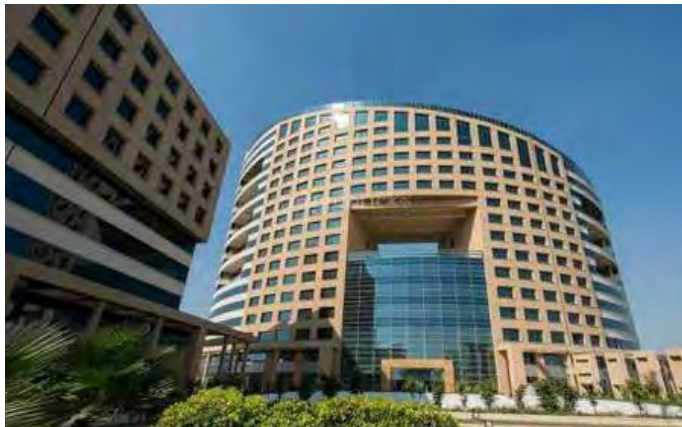
Corporate office in Gurgaon (Source: https://worldarchitecture.org/architecture-projects/hggvh/cyberwalk-2c-manesar-project-pages.html )
