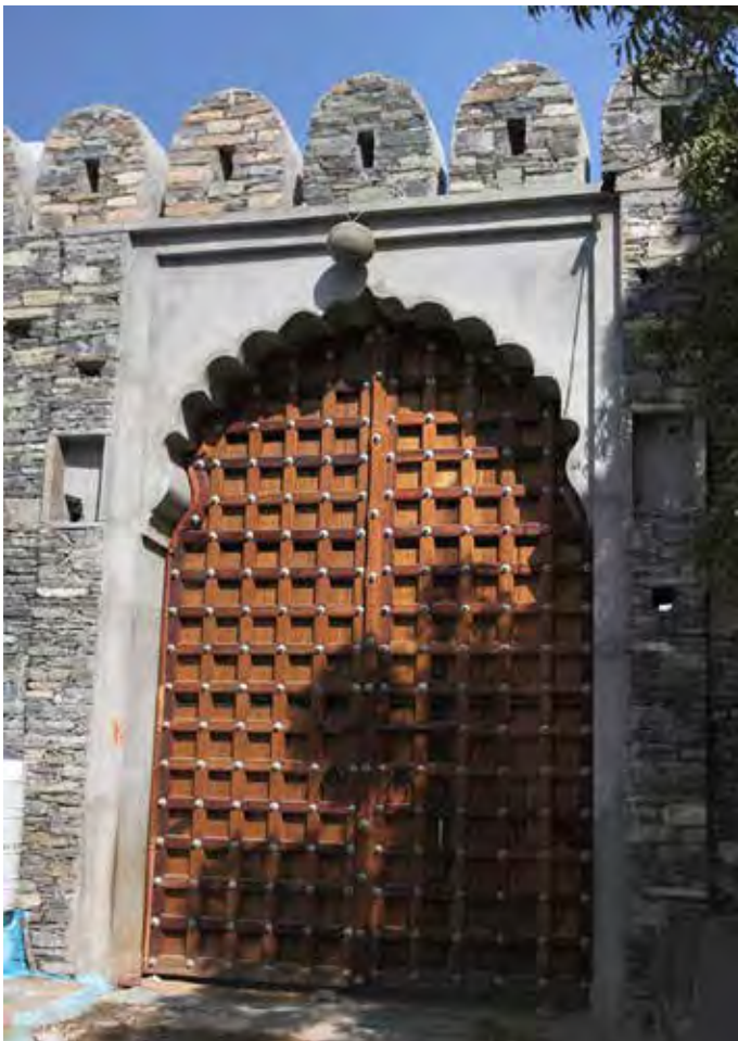
Figure 15: Design Implementation of Gate (after)
