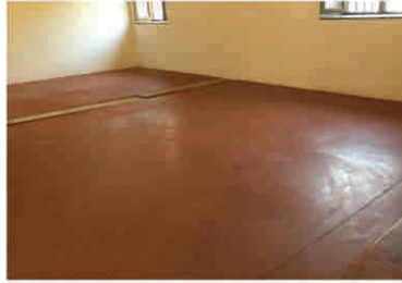
Flooring inside after restoration
