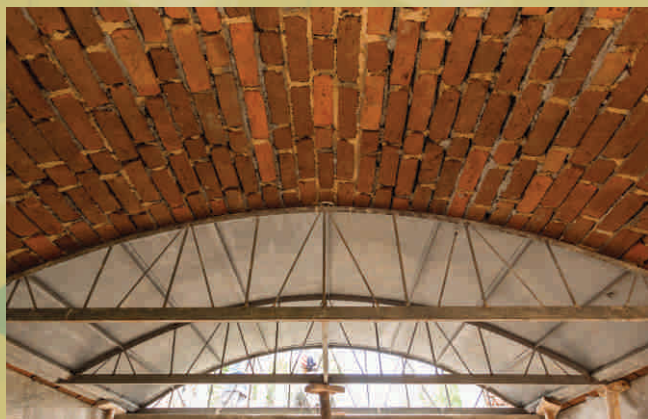
Figure 8: Segmental vaulted roofing in bricks
