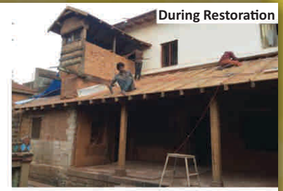
Rear Court Verandah
