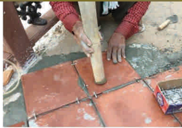
Flooring being done in Balcony
