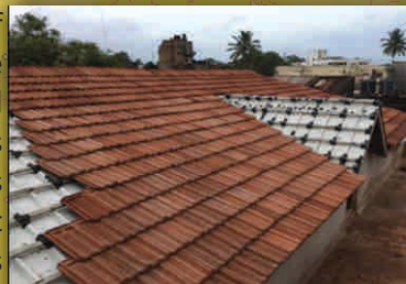
Terracota Tiling in process over main roof
