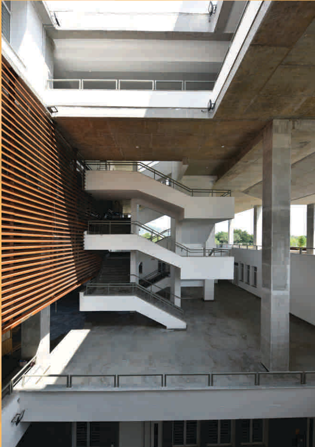
The double helical staircase connects alternate planes
