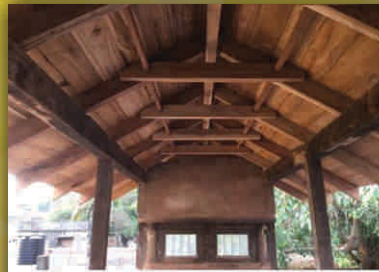
Wood work for Roofing
