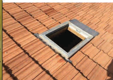
Skylight taken from Top Second Floor
