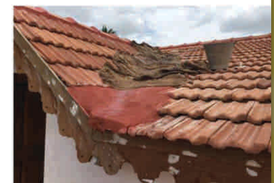
Valley - Terracota tiling over main roof
