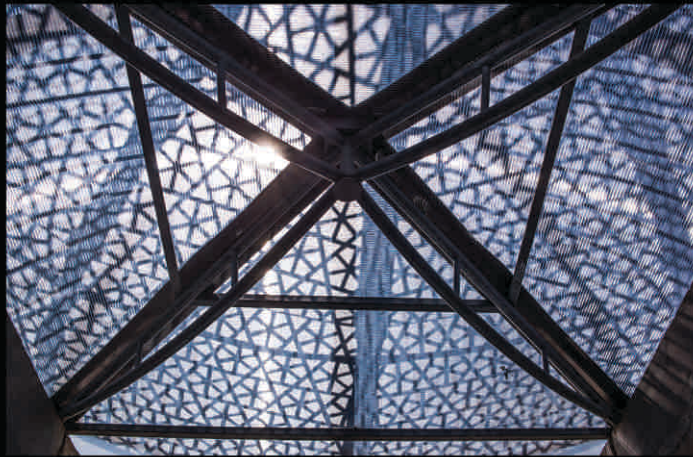
Metal screen used on the dome to keep the transparency and clarity in design
