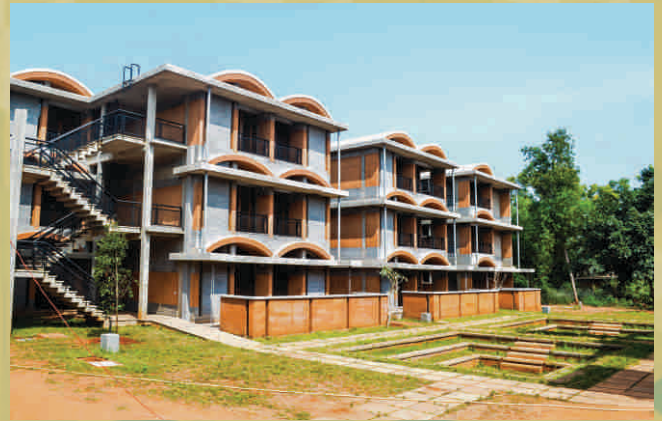
Figure 2: Central plaza roof water harvesting
