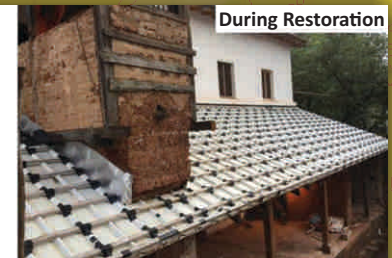
Laying of TRIMDEX over wooden boardings
