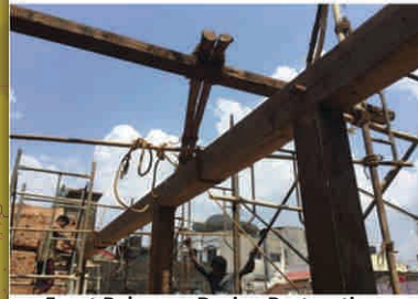
Front Balcony - During Restoration
