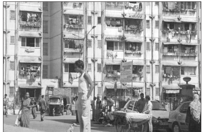
Slum Resettlement Under Mumbai Urban Transport Project with 225 sqft Dwelling Units
