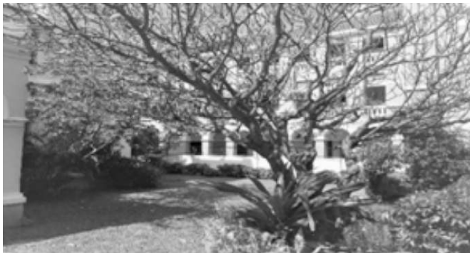
Well designed built environments can enrich the learning : open courtyards and deep colonnaded corridors, renovation and redesign of a century old High School in Chennai
