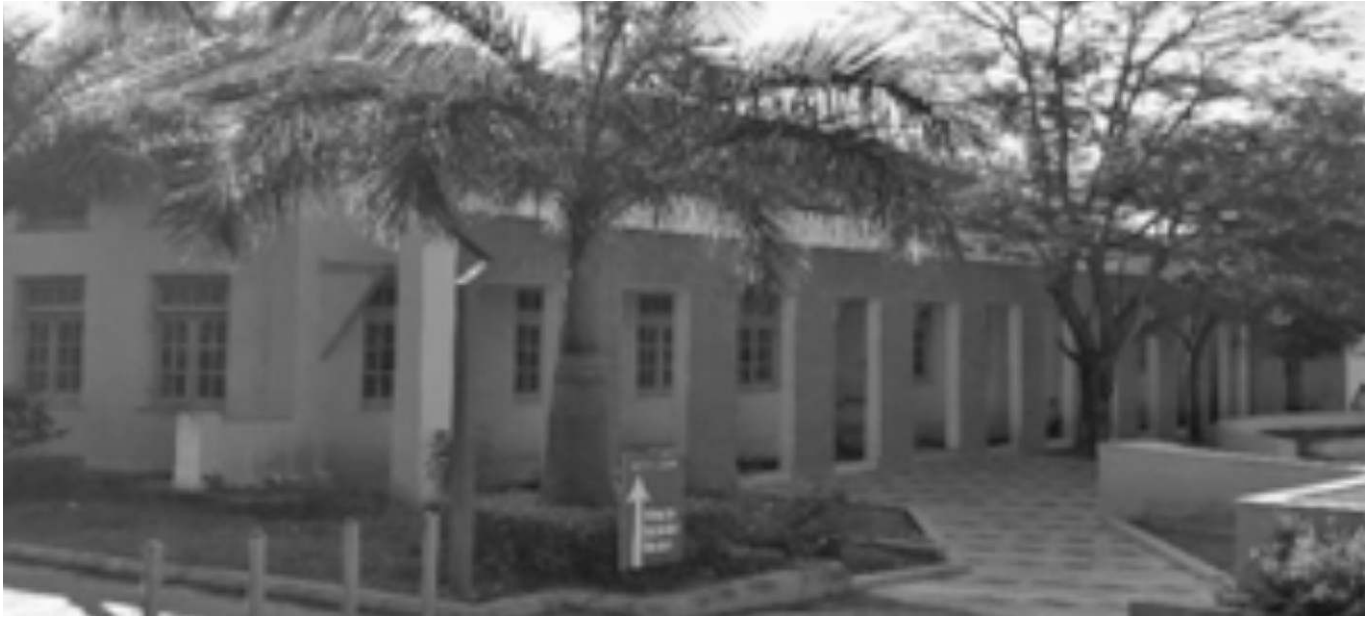
A climate sensitive façade improvement to an Engineering college laboratory - Hubballi, Karnataka
