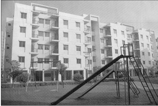
Shukhobrishti at Rajarhat New Town, Kolkata, developed by Shapoorji Pallonji in association with the KMDA and West Bengal Housing Infrastructure Development Corporation (WBHIDCO). The project covers 150 acres of land in Rajarhat and has 20,000 dwelling units: 10,444 (LIG) apartment with carpet area of 320 sq.ft., 3840 MIG apartments of 480 sq.ft. and balance 5716 apartments, each having an area of 690 sq.ft.
