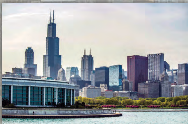
Figure 1: Willis Tower formerly known as Sears Tower designed by Skidmore, Owing and Merrill in 1973
