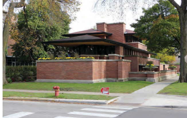
Figure 13: Robie House, a masterpiece of the Prairie style and a forerunner of modernism in architecture, Frank Lloyd Wright broke down old barriers, creating a residential design with a horizontal roofline, large overhanging eaves, continuous ribbons of windows, and a wide-open living space at its center.
