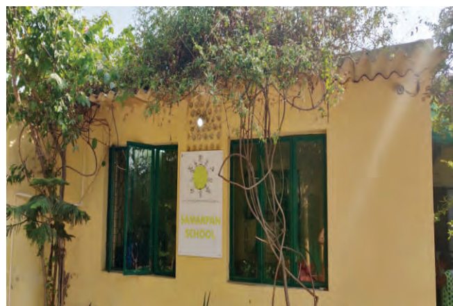
Figure#6 (a) (b) (c): Samarpan School construction details and facade (Source : Youtube and Author)
