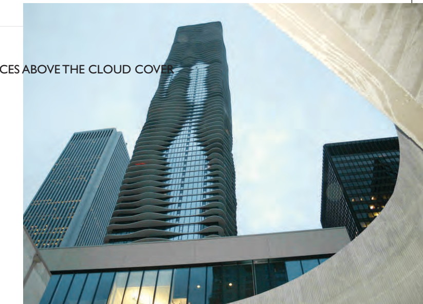
Figure 8: Taking inspiration from striated limestone outcropping – a common feature in the Great Lakes region – the façade of Aqua Tower undulates in and out. Floor slabs across the height tower vary according to use, views and sunlight creating an undulating and sculptural elevation.
