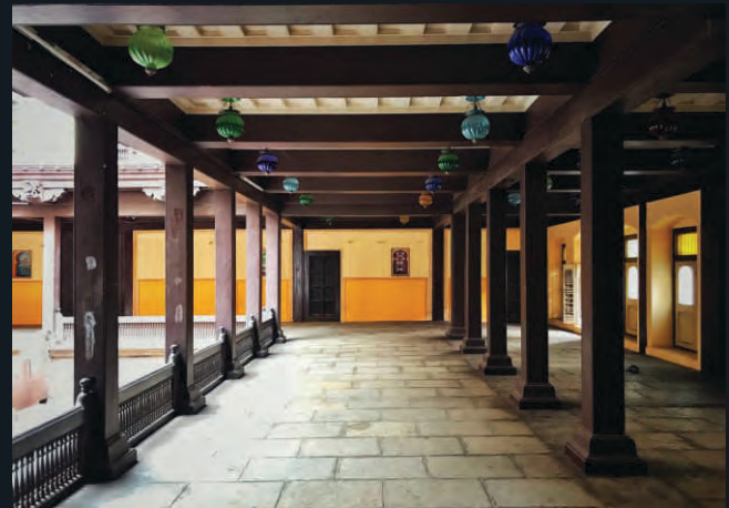
Fig.#3: Pictorial example showing chowk of Vishrambag wada, Pune situated in heart of city.
