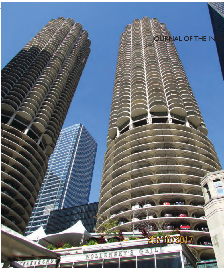
Figure 9: Designed by Bertrand Goldberg way back in 1964, Marina Tower, with its iconic corn cob towers, and identical floor plans, became the first circular apartment buildings in history. It was designed as a self-contained town, full of residential and commercial units – a revolutionary concept at that time. Goldberg then went on to continue designing many iconic building residential towers like the Old Prentice Women's Hospital and Stony Brook University Hospital in Chicago.
