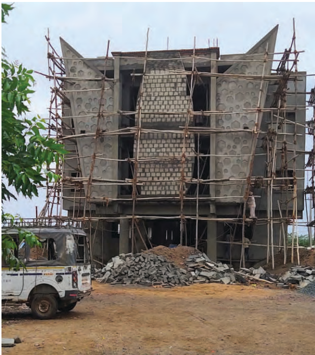
Figure#9: Construction in progress - Stage #3
