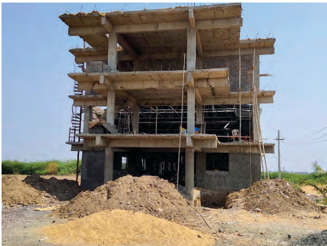
Figure#10: Before Construction of Curved body and wings
