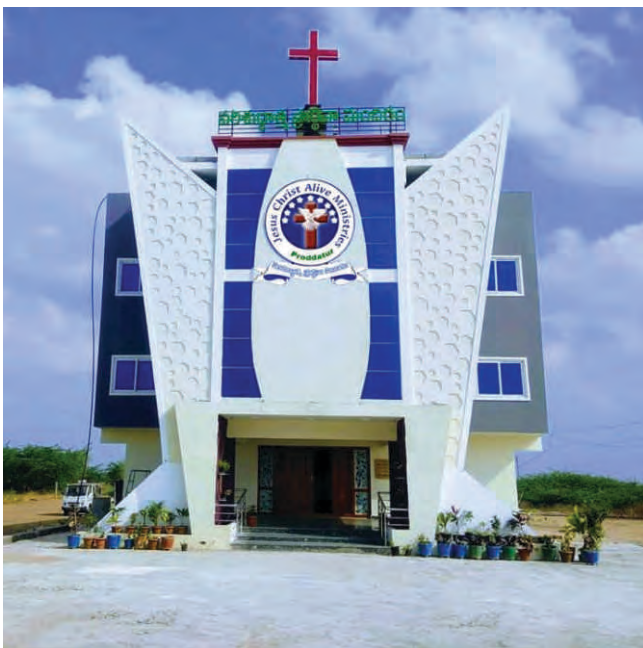
Figure#13: Final finished elevation - front view
