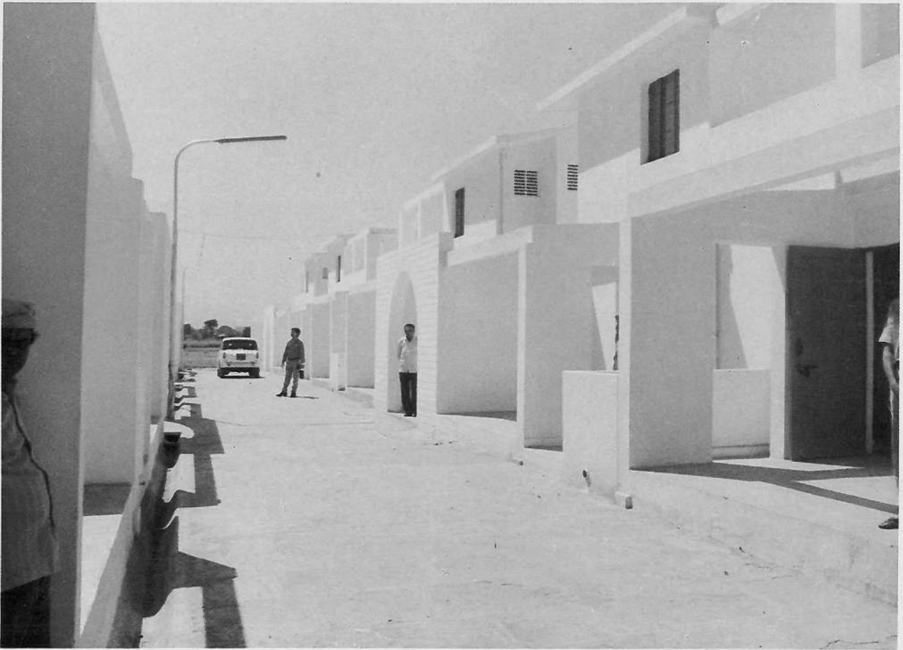
Roadside view of cluster
