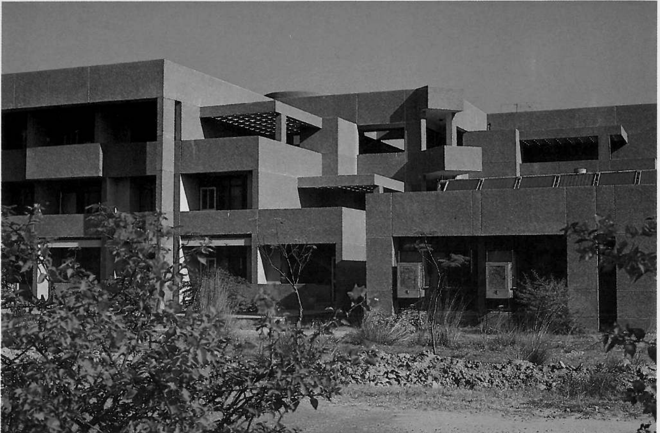
Post Graduate Students' Hostel— Corner details and terraced construction.
