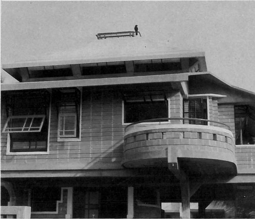
Facade with a curved balcony
