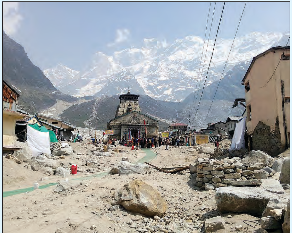
Picture 1 : Shows front side of the Temple and path towards the temple and damaged surrounding structures.
