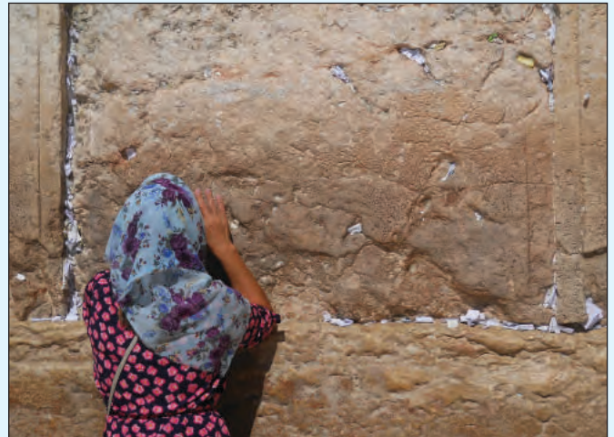
Stories in a crack Western Wall
